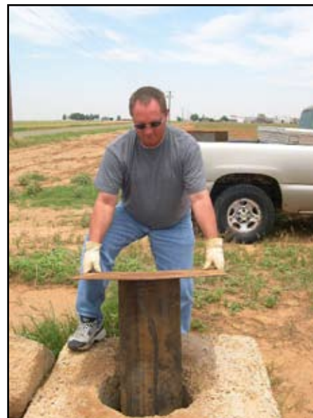
Installing a well plug
